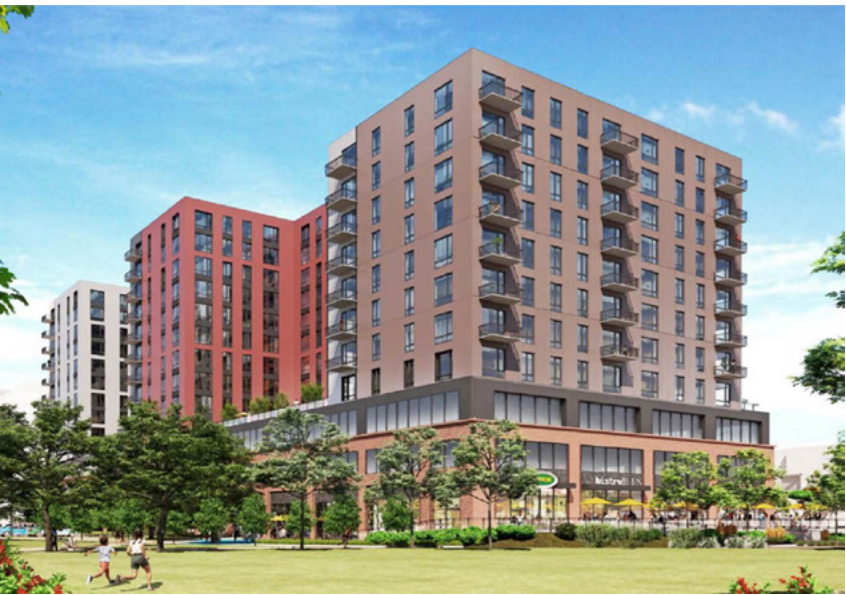
Cambridge Point campus, residential tower, view southeast toward Fawcett Street.
