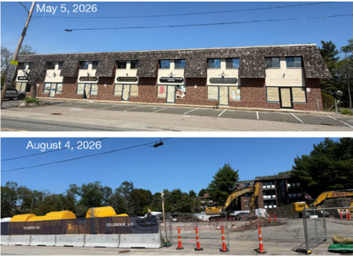
87-101 Blanchard Road, former commercial building, view from Hamilton Road.
