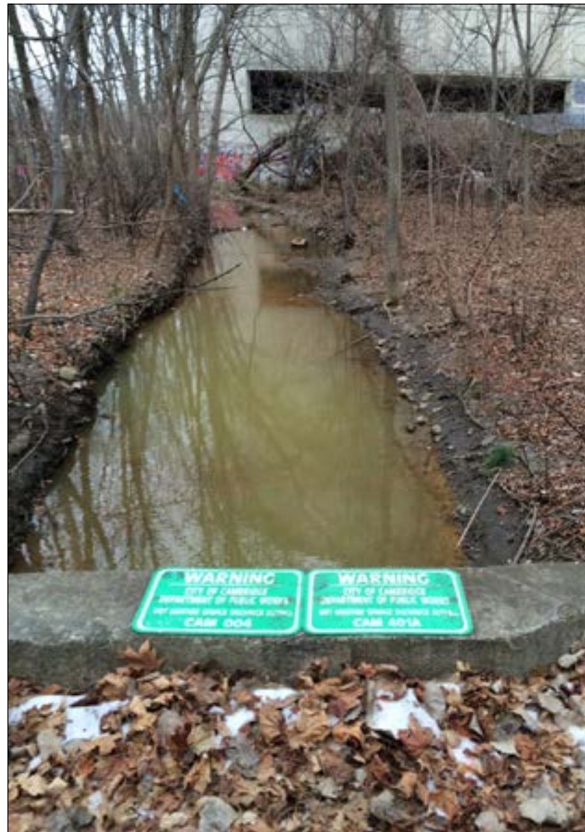
An Alewife Brook combined sewer overflow outfall in 2016.
