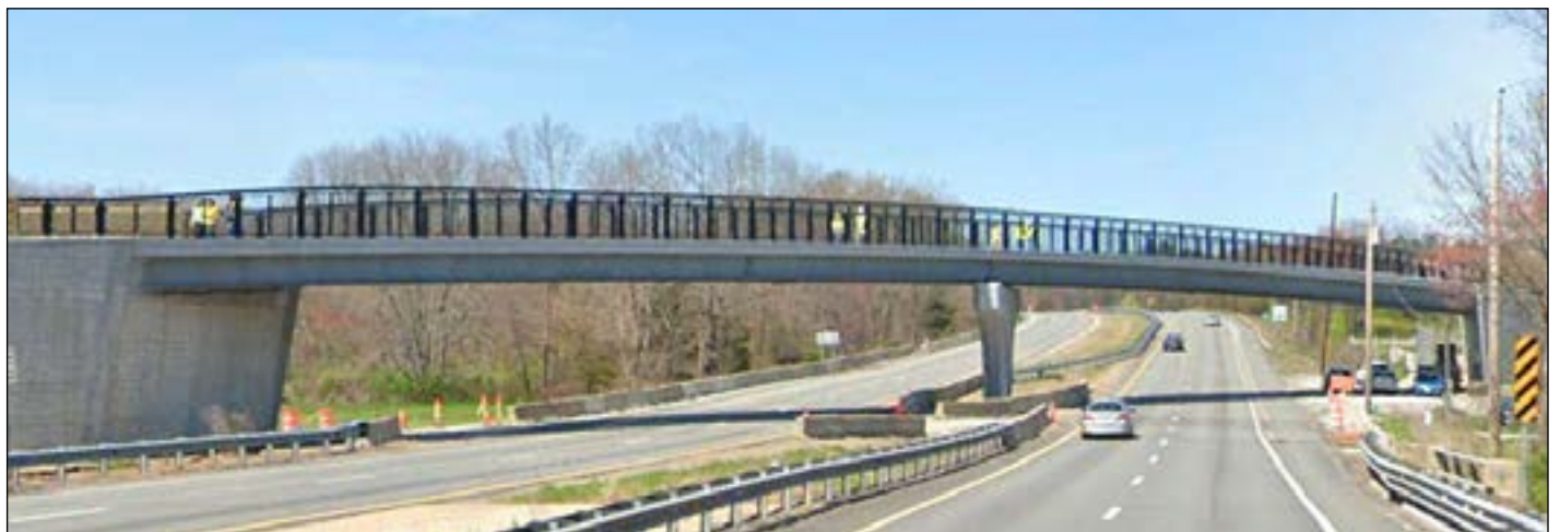
The Bruce Freeman Rail Trail bridge over Route 2 in Concord.
