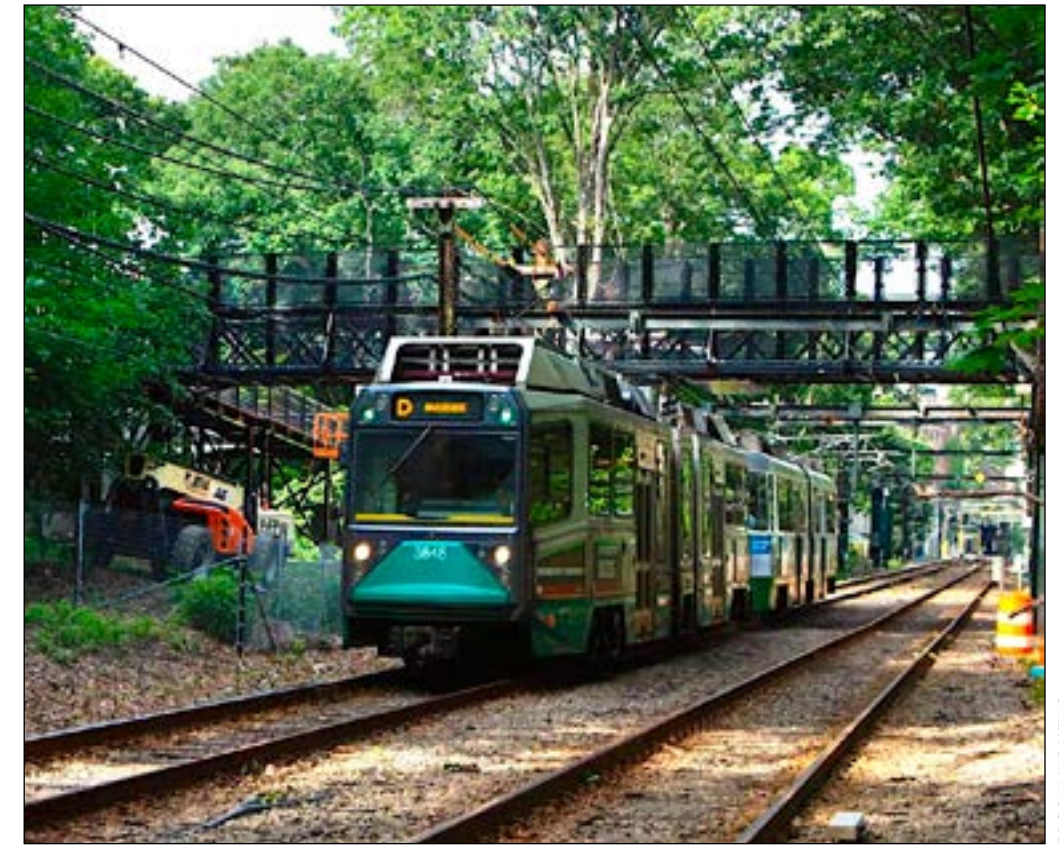
Carlton Street footbridge, Brookline.
