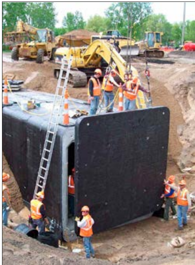
"Cut and cover" tunnel construction.
