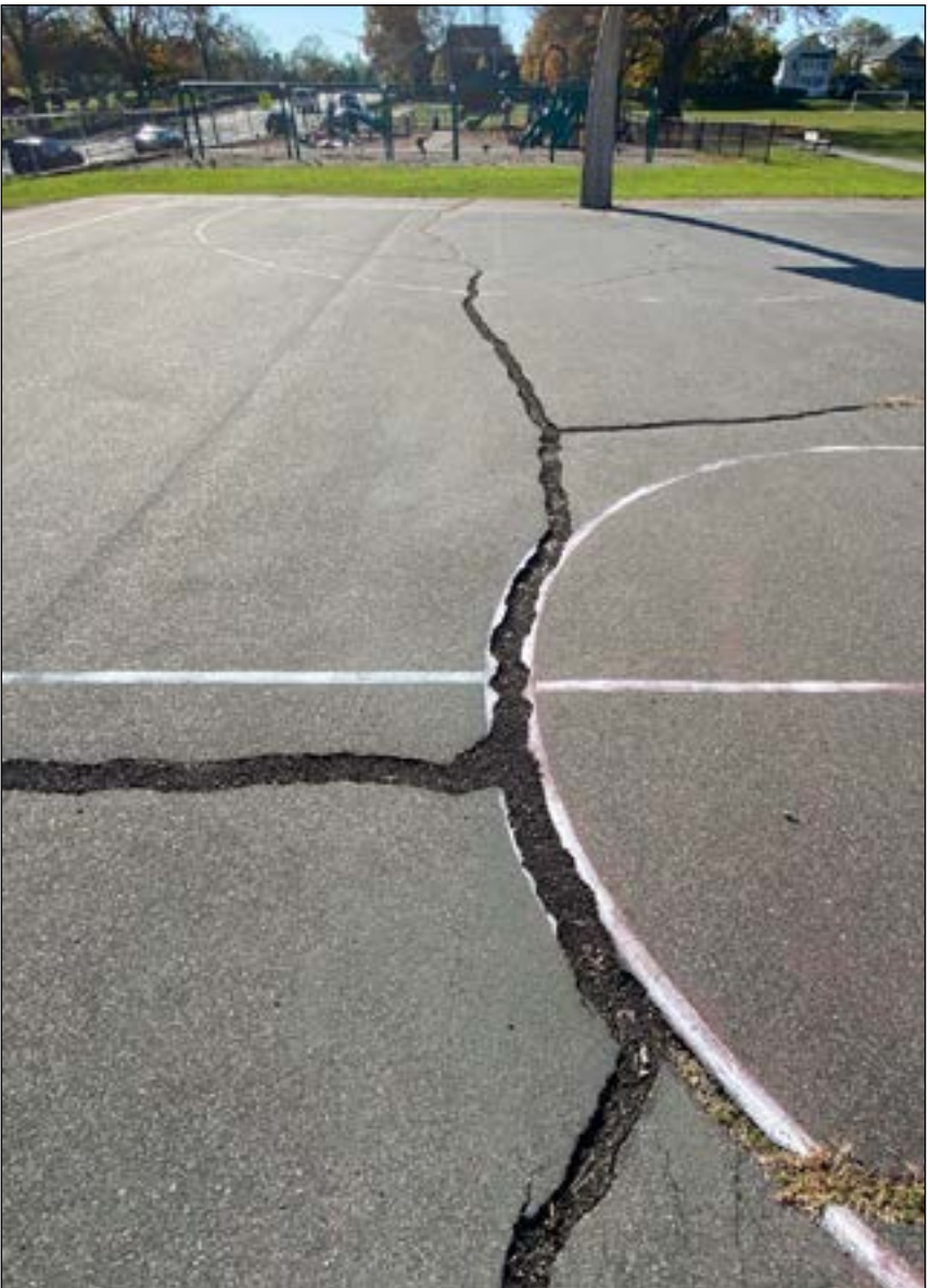
Cracks in the Grove Street Playground pavement.
