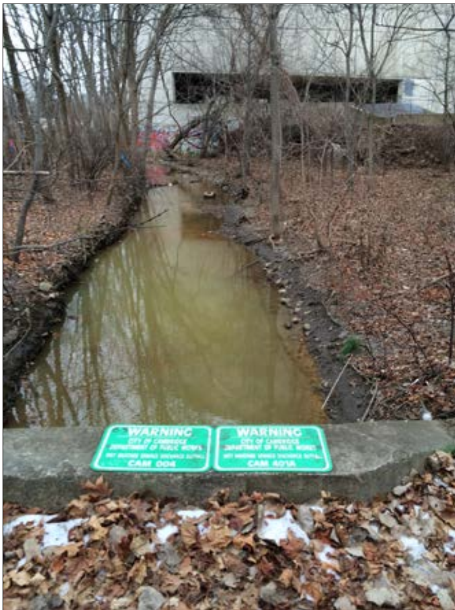
An Alewife Brook combined sewer overflow outfall with warning in 2016.
