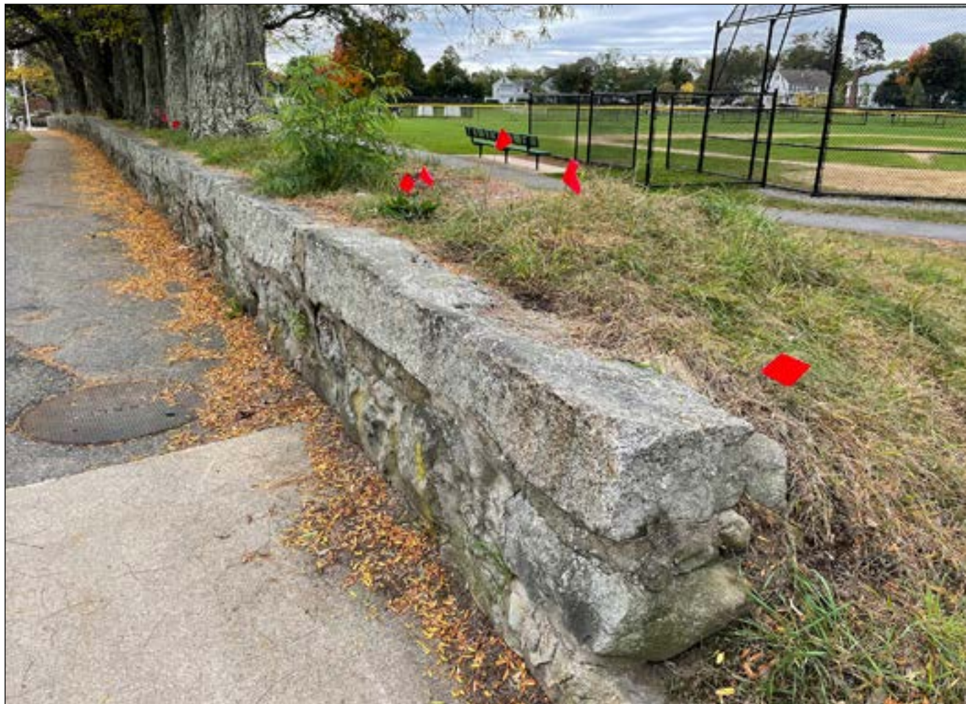
Flags indicating rodent treatments at the corner of Grove Street and Grosvenor Road.
