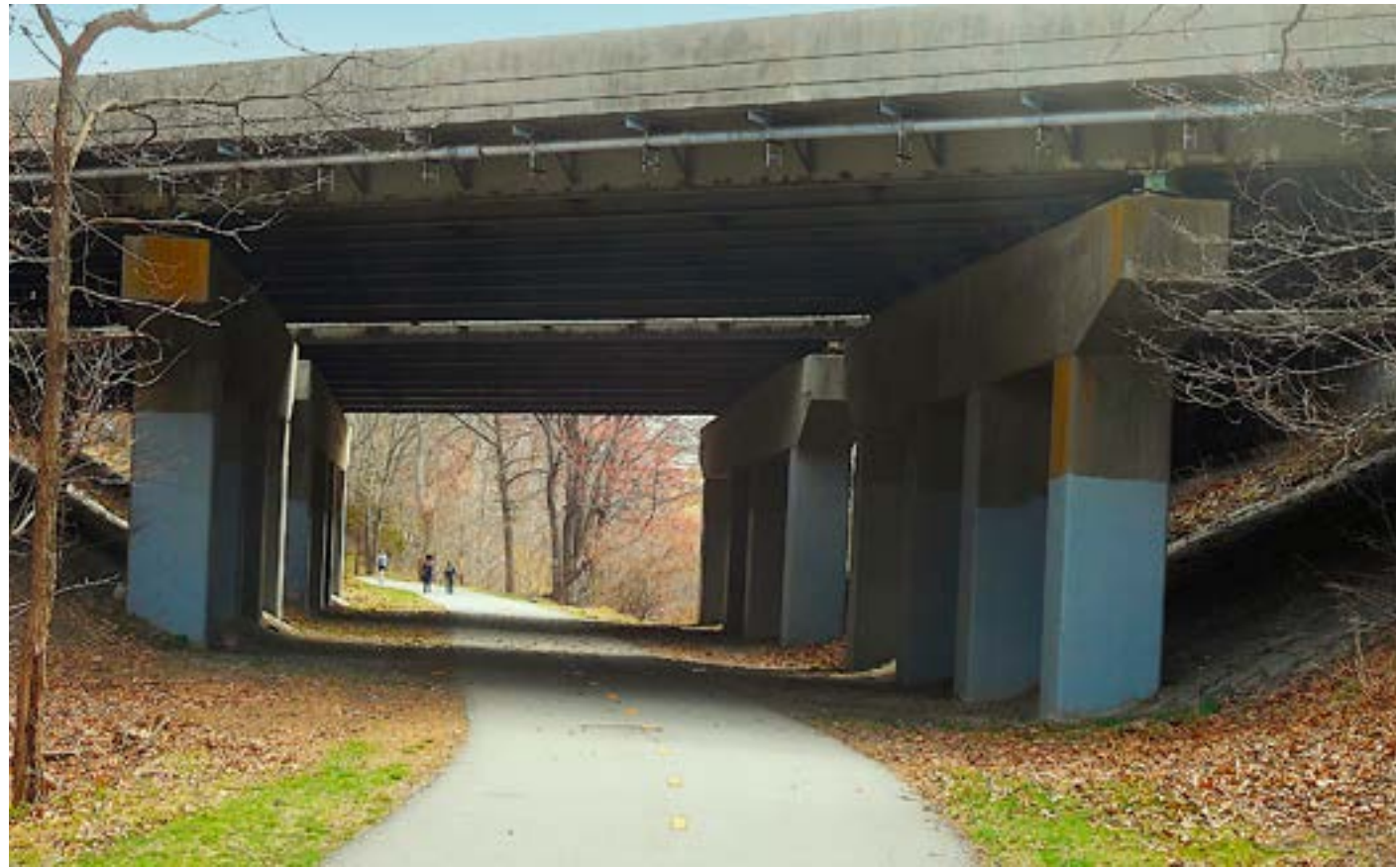
Mass Pike underpass, Cochituate Rail Trail.
