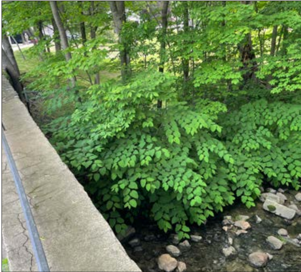
Knotweed thriving at the Common Street bridge.
