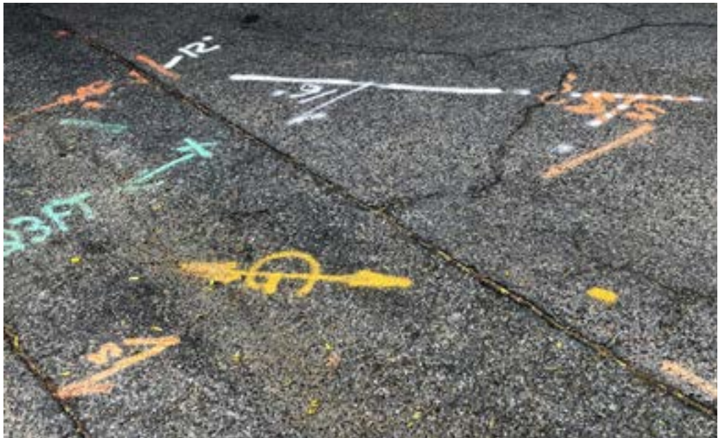
Road markings for sewer work.
