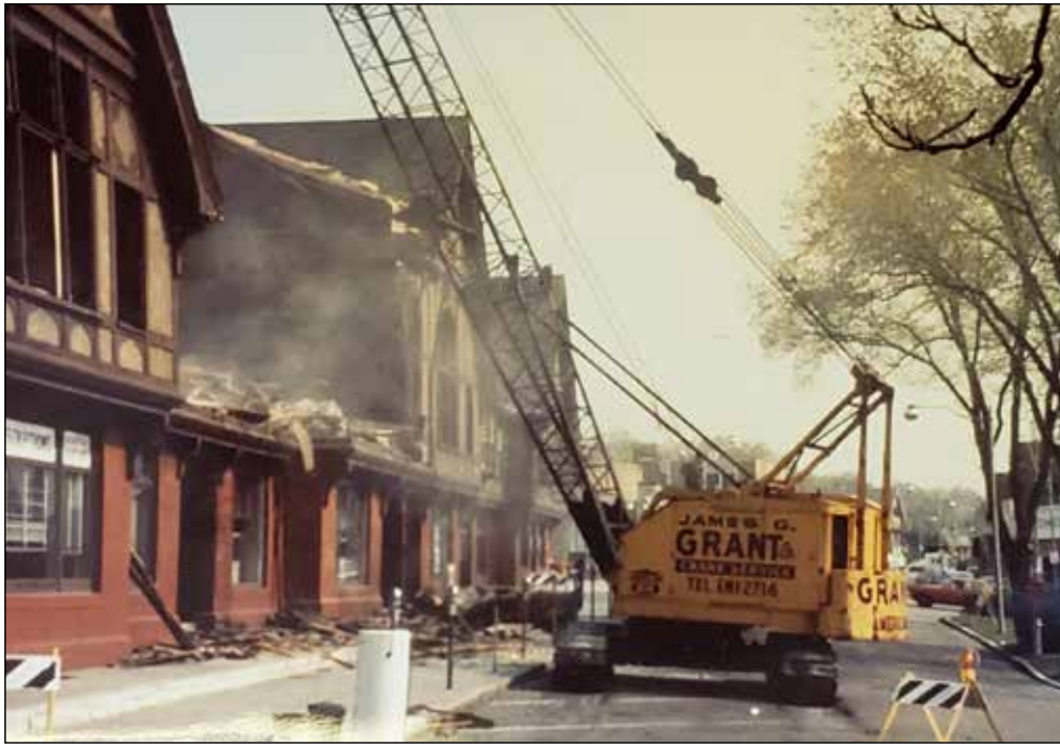
Demolition of Belmont Center's Olive Block in 1968.
