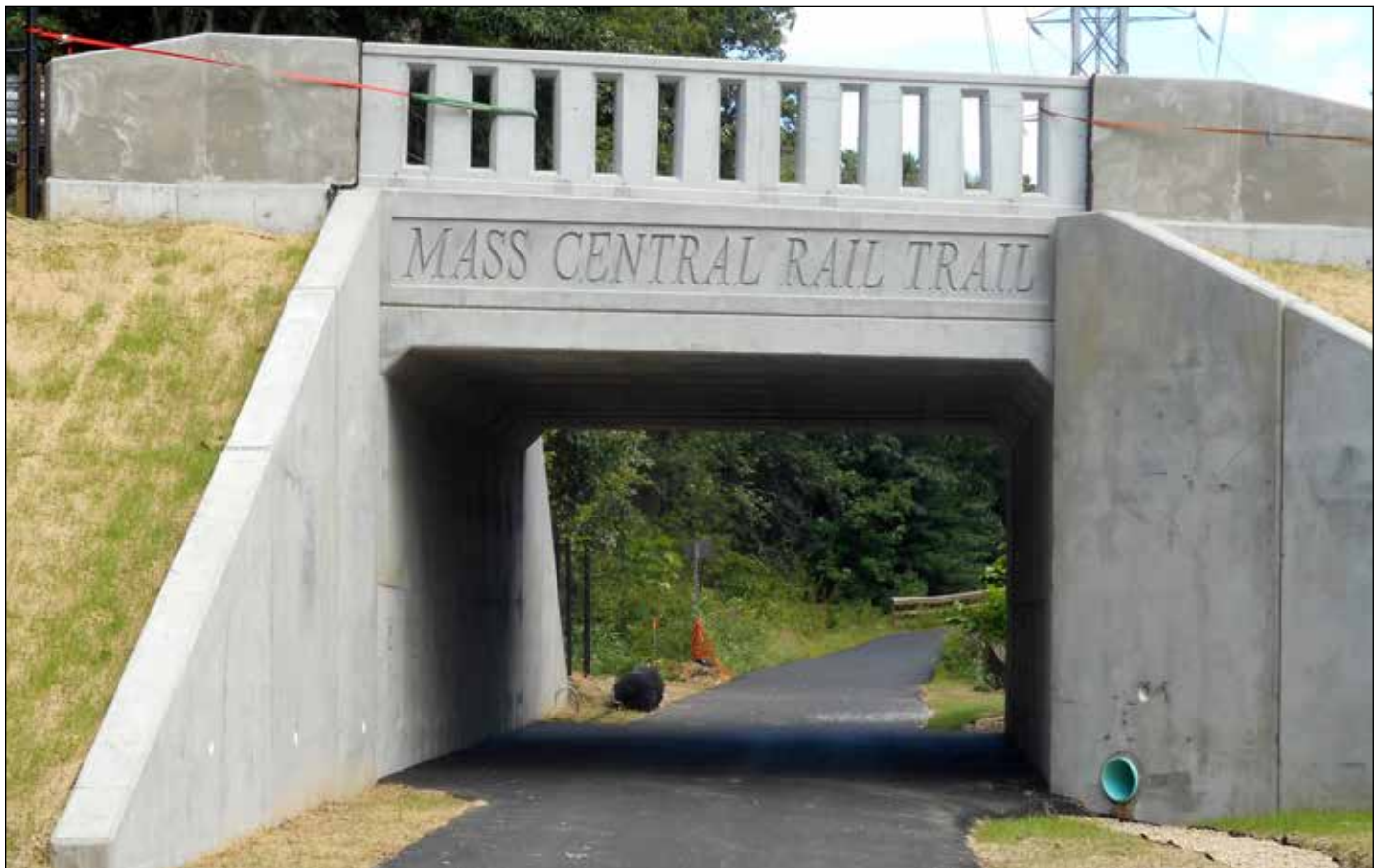
A view of the new Conant Road Overpass, Mass Central Rail Trail, Weston.
