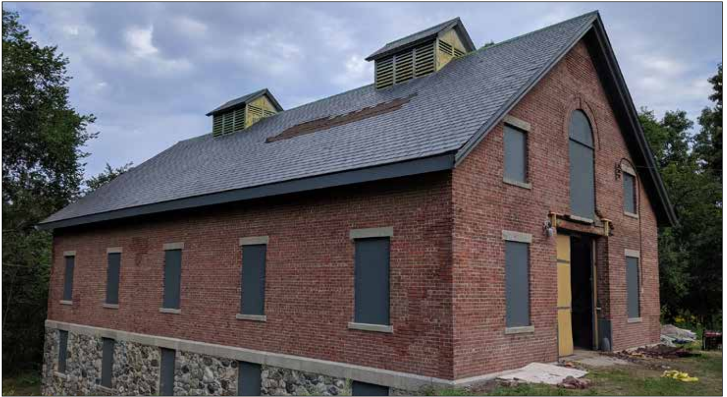
The cleaned and stabilized McLean barn, left side.
