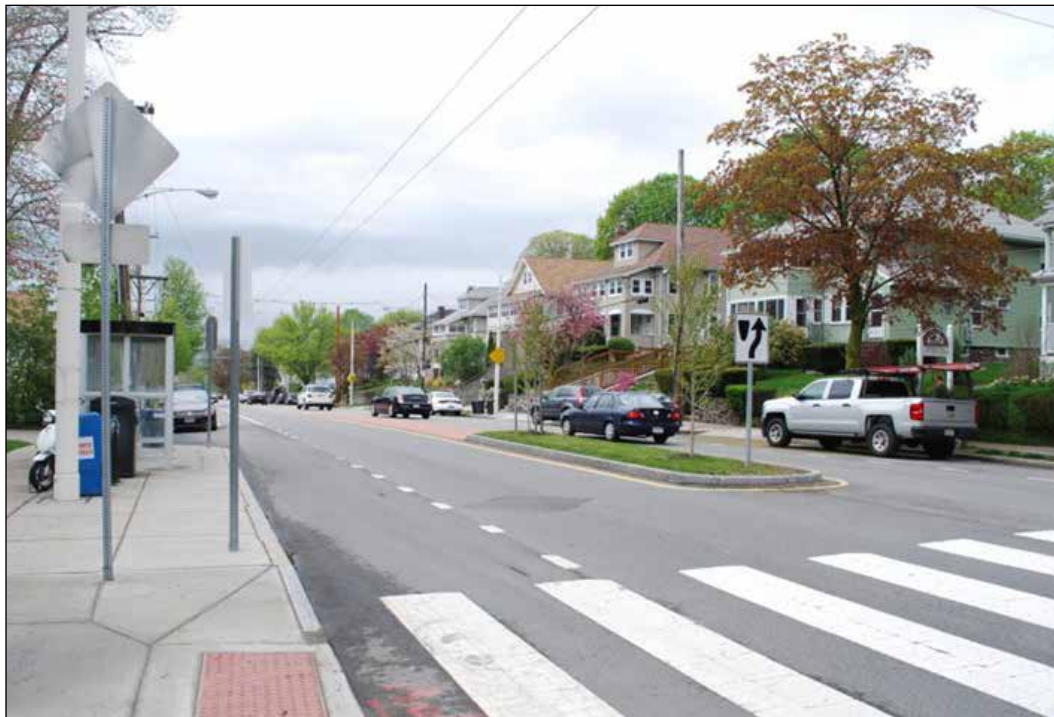
Pedestrian-oriented streets: Trapelo Road at the corner of Williston Road in Cushing Square has a center divide, clear bike lane markings, enlarged crosswalk, newly paved and expanded sidewalk, and a covered bus stop.
