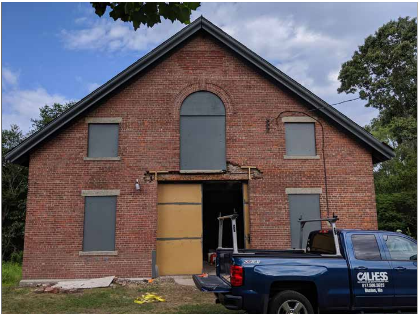
The McLean Barn front after cleaning and stabilization.
