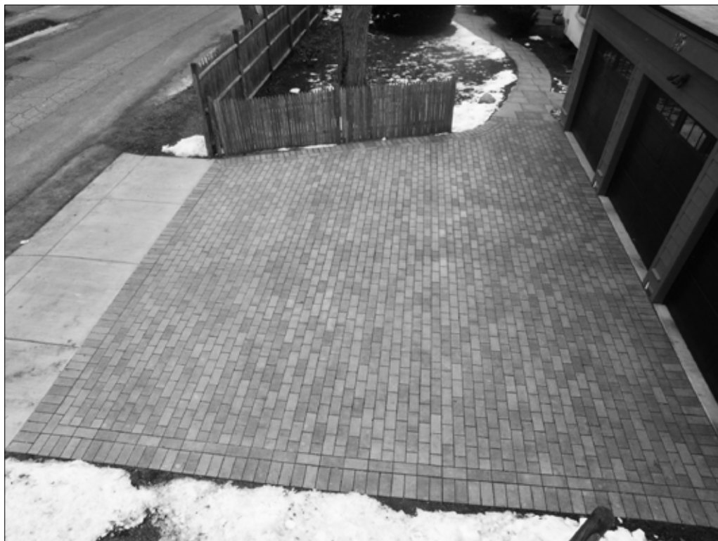
The Lenk/Kossak completed permeable driveway.
