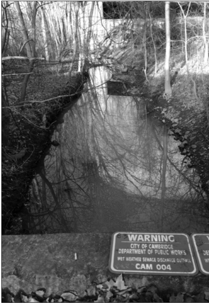
The CAM004 combined sewer overflow.
