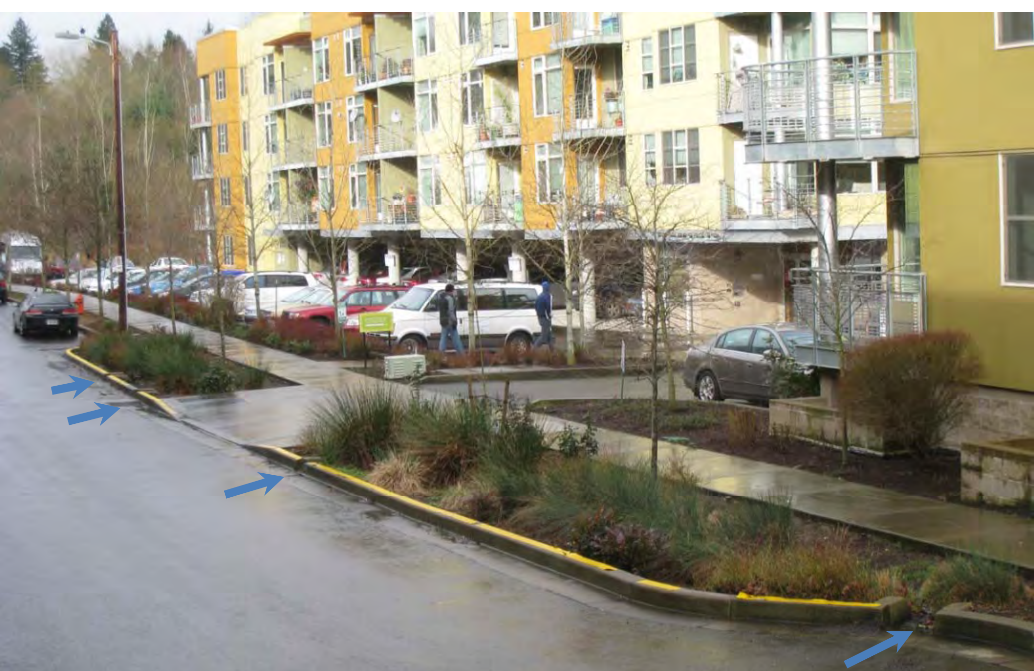
Bioretention Basin: Green Street Application Curb Extension, Portland OR
