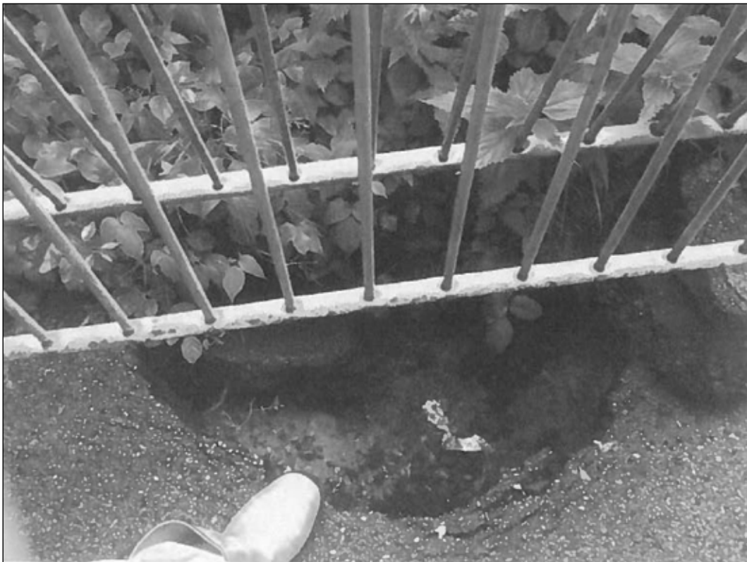
Sinkhole in the Duck Pond dam.
