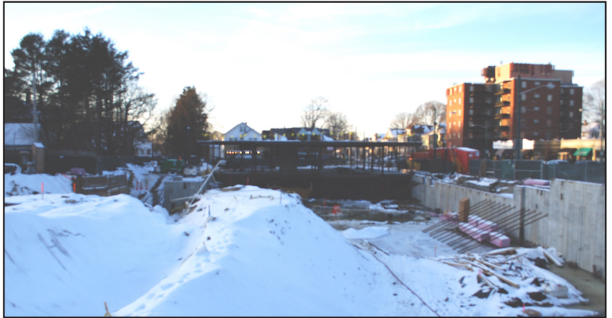
Looking at the Bradford construction site from Common Street, the mound in the center is where the contaminated soil is piled.
