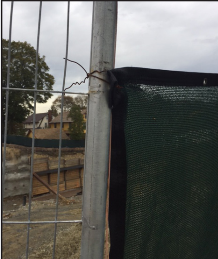
One example of flimsy, unsafe fencing at the Bradford: a piece of canvas held by a single strand of poorly wrapped wire. (See story on page 11.)
