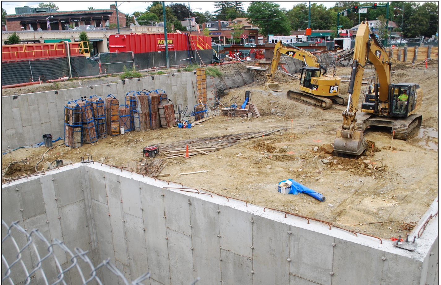
At the foundation work for the Winslow building, at the corner of Williston Road and Trapelo Road, the crew continues to remove stubborn ledge so they can lay down the cement floor of the parking garage.
