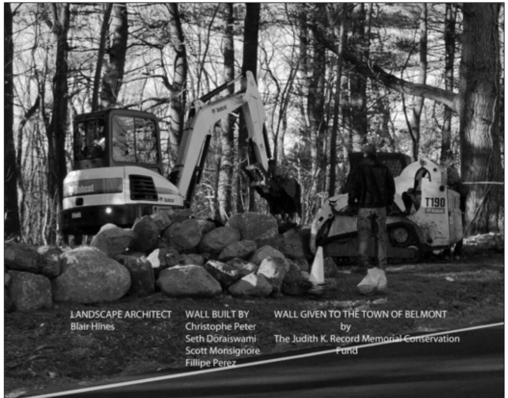
An historic stone wall on Concord Avenue was rebuilt using Judith K. Record Fund monies.
