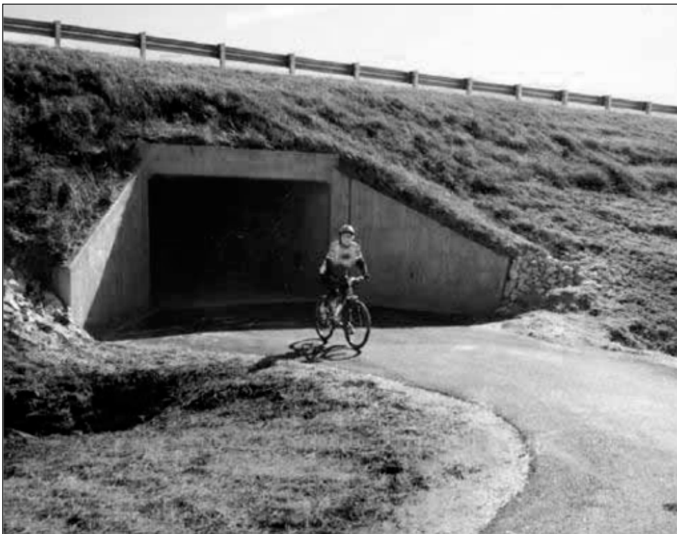
A community path underpass.
