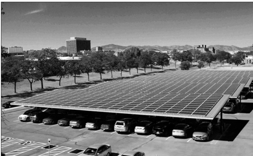
The future? Solar-panel-covered parking, Denver Federal Center, Denver, CO.
