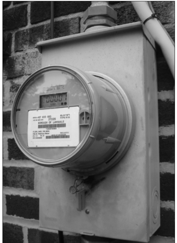
A Smart Meter.
