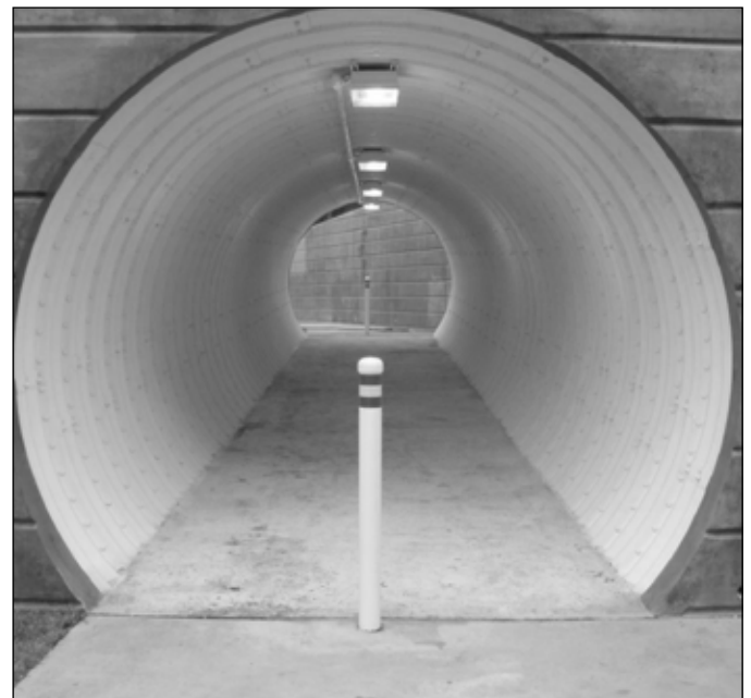
The completed Tallahassee pedestrian tunnel.
