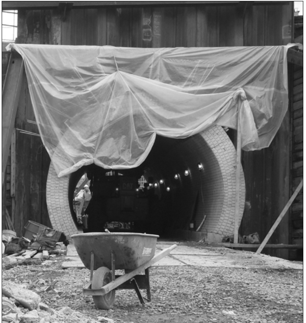
The Malvern, Pennsylvania, pedestrian tunnel under construction.
