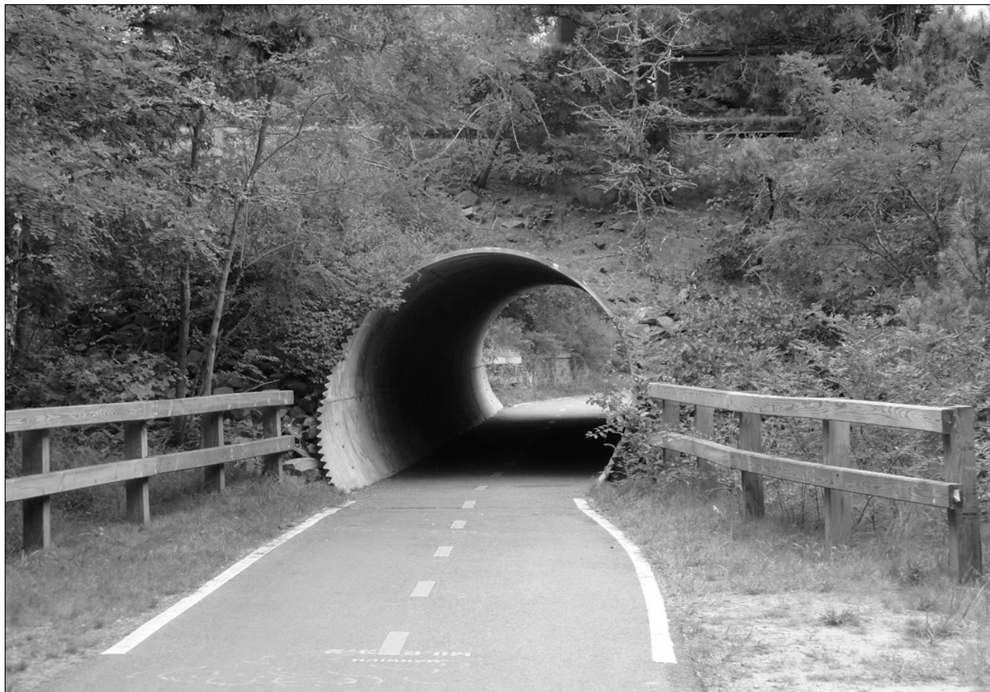
Tunnel on the Cape Cod Rail Trail.
