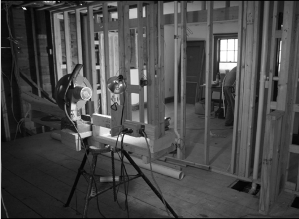
Brownsberger's home was stripped down to the studs.
