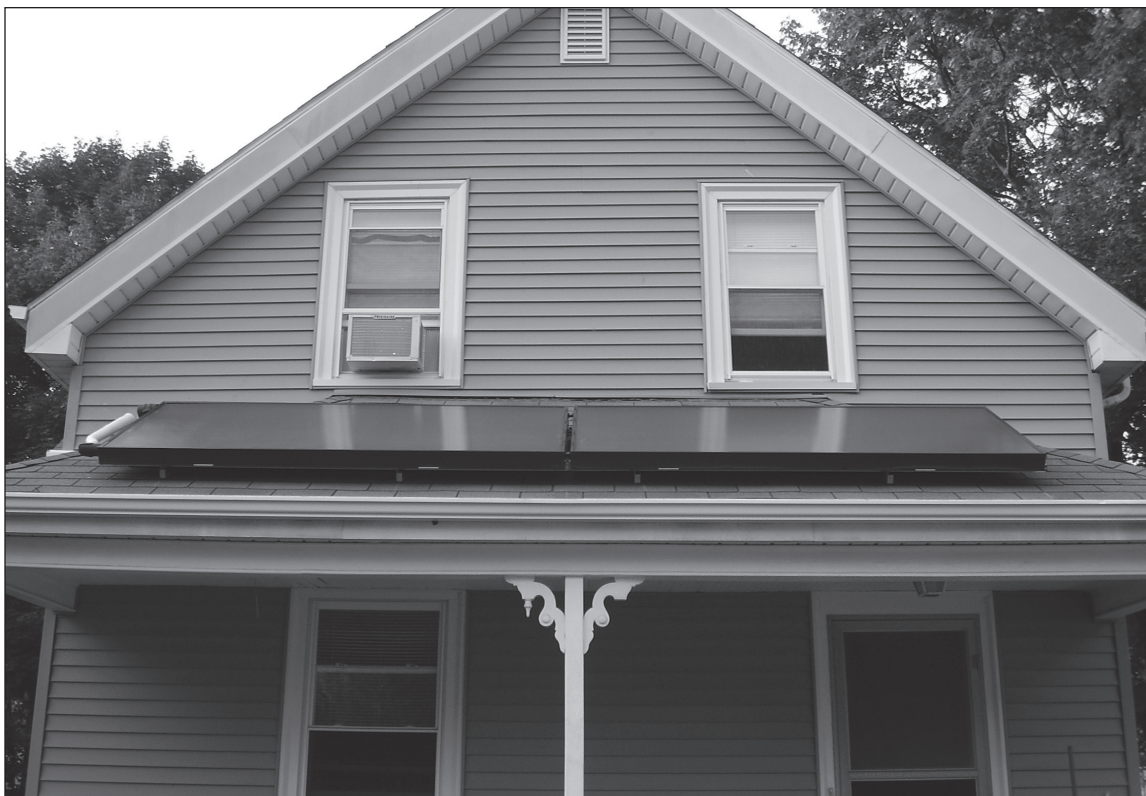
The final installation.
