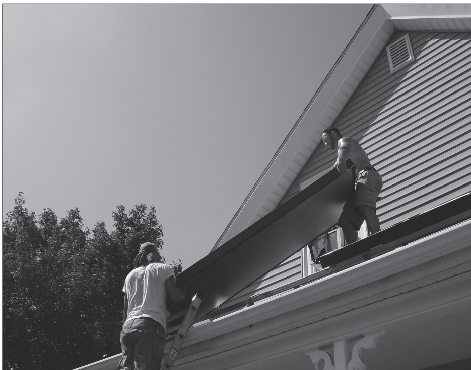
Solar panels are lifted to the porch roof...
