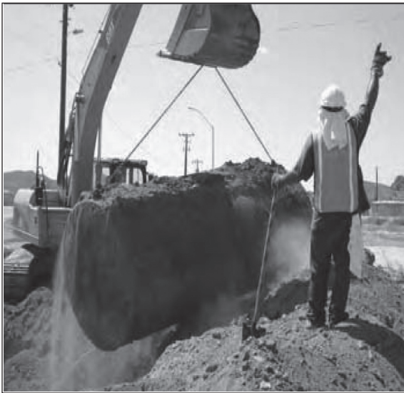
An underground storage tank being removed.
