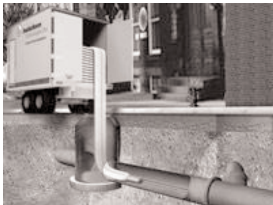
2. Next, hot water or steam is used to cure the resin and form a tight-fitting, jointless and corrosion-resistant replacement pipe.
