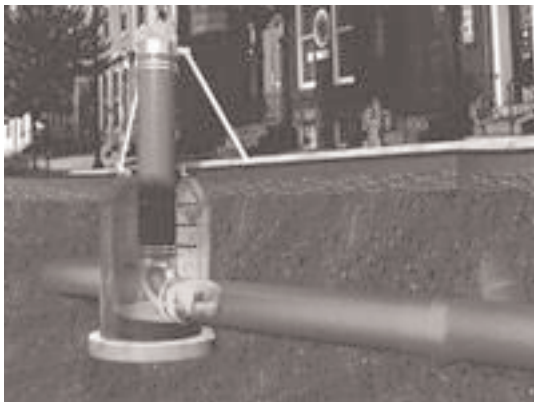
1. A resin-saturated, coated felt tube is inverted (left) or pulled (right) into a damaged pipe.
