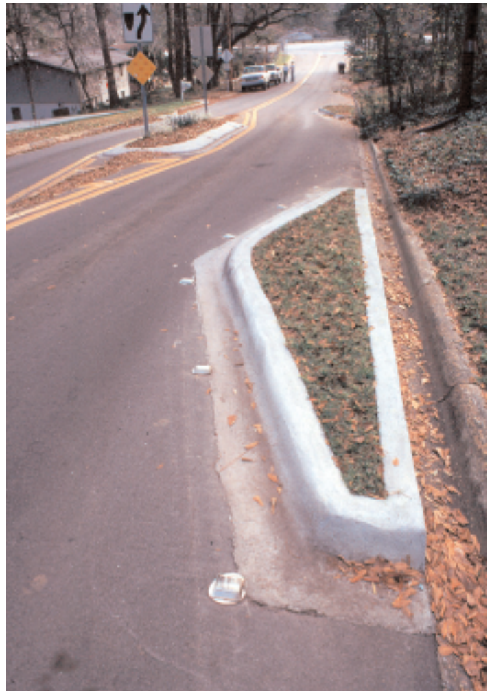
An example of a chicane, a traffic-calming device.. Used with permission www.pedbikeimages.org / Dan Burden
