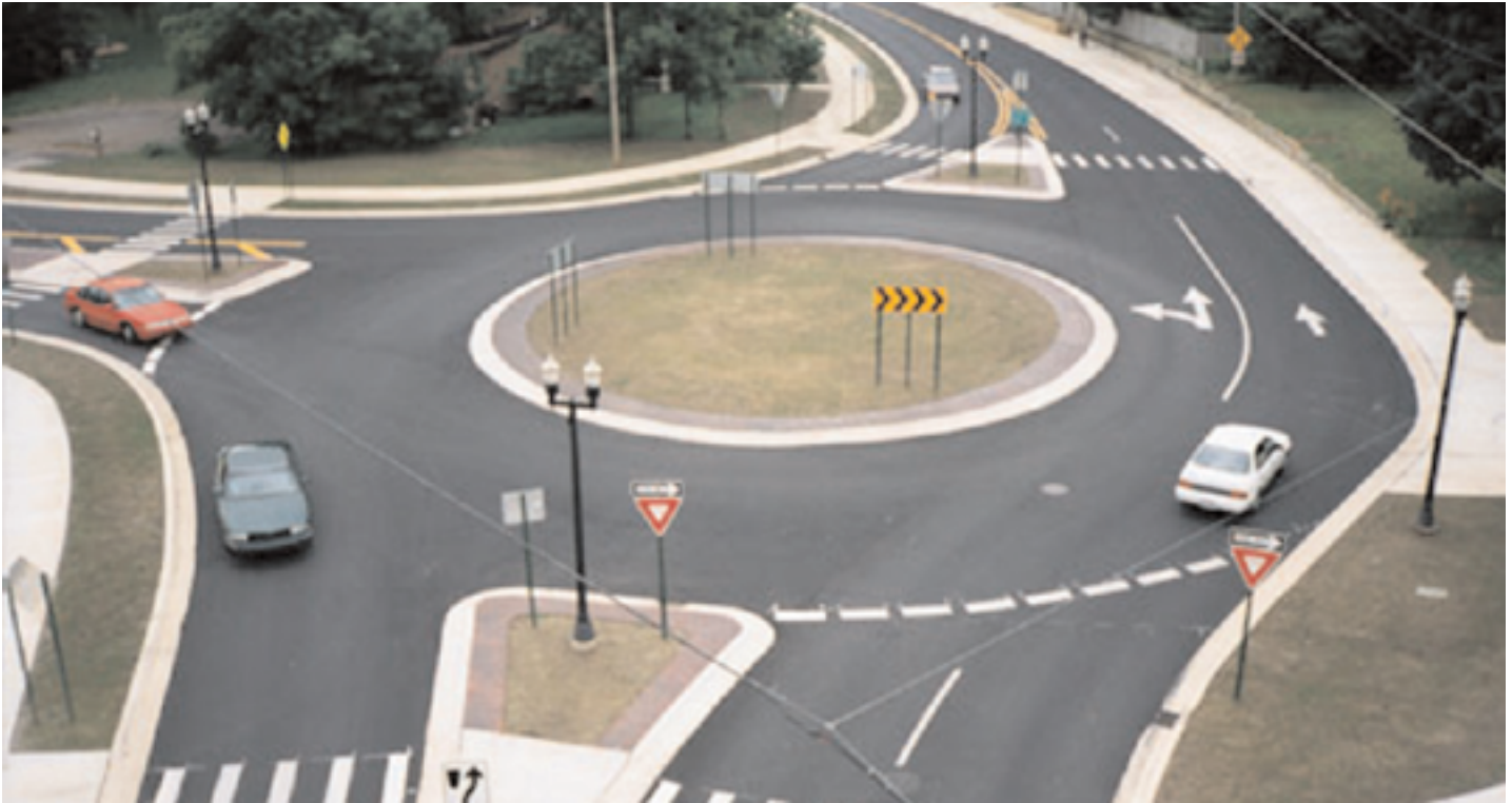
A roundabout has four crash pints, rather than the 16 found in rotaries. Used with permission www.pedbikeimages.org/Portland Office of Transportation .
